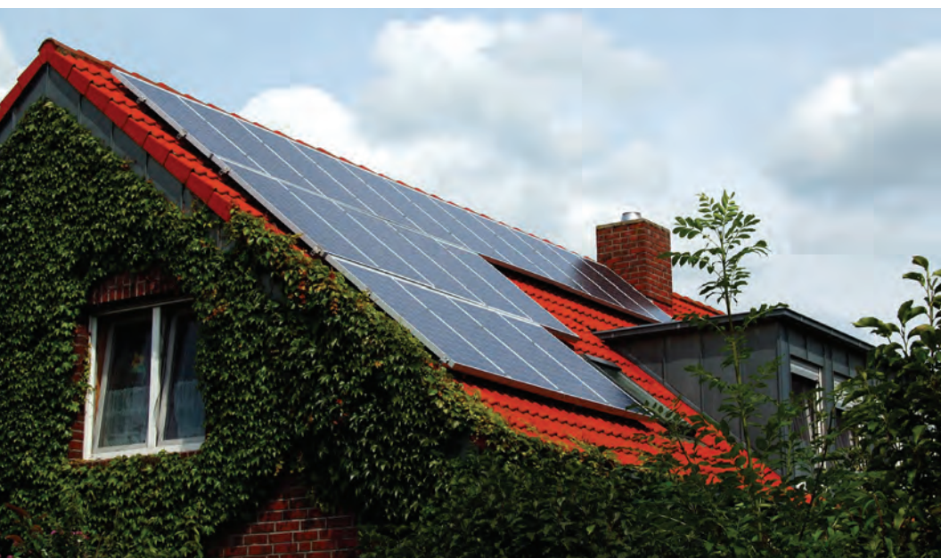
SOLAR PANELS installed on a residential roof
